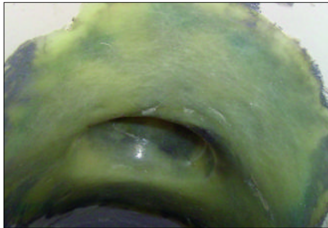
Typical installed Top Hat lateral seal.
